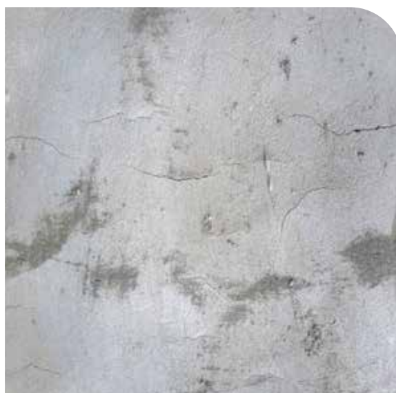
Blistered and cracked wall surface due to application of non-compatible mortar directly on AAC Wall surface
