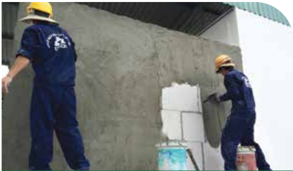
Plastering using EBP -202 EBLOCK Mortar
