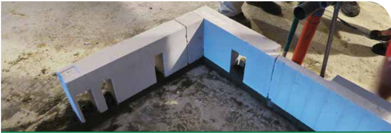
Apply waterproof block EBLOCK EBW at base-course in WC
