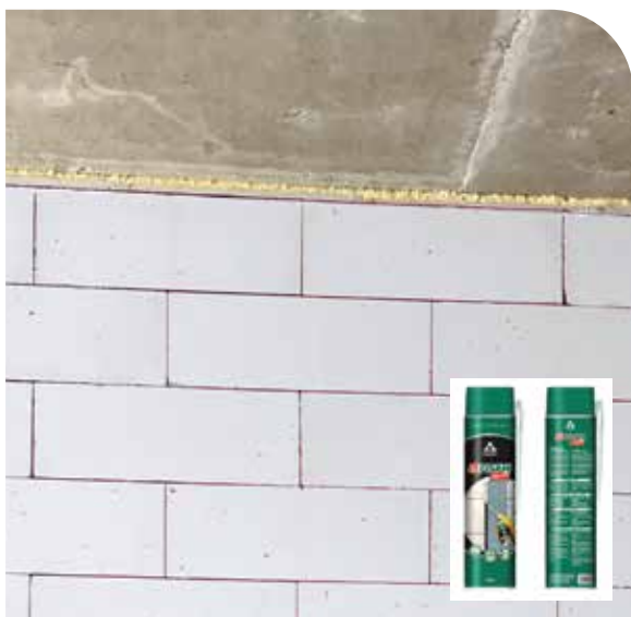
Filling gaps and joints with PU foam or other compressible materials
