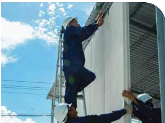
Contracting team to install EBLOCK panel vertically
