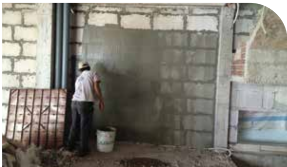
Normal cement-based mortar application on the surface of Primer Mortar EBH-401
