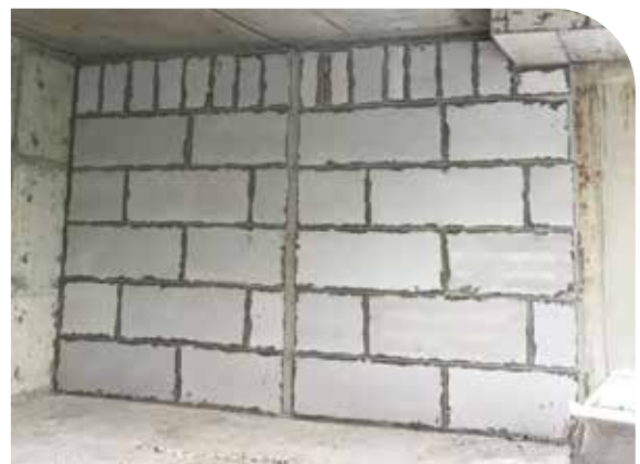
Short Panel of 1.5 meters installed horizontally
