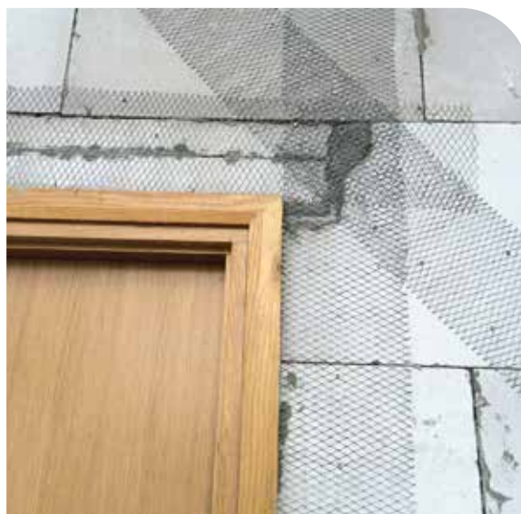
Apply reinforced net at door and M&E groove location
