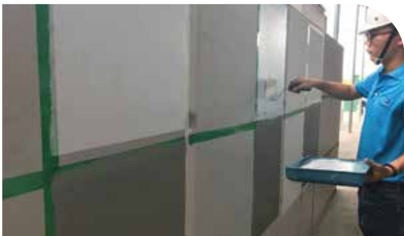
Finish Coatings application on EBS-300 skimcoat surface (without putty layer)
