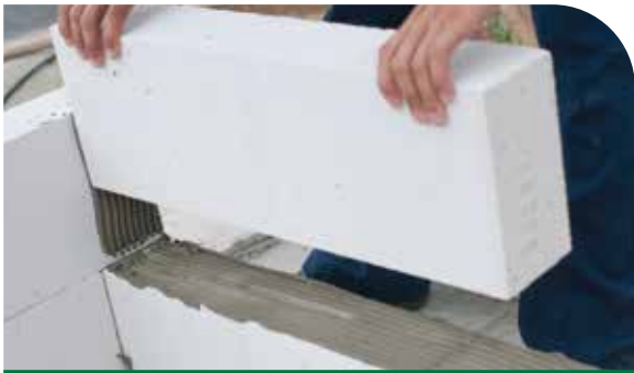
Thin-bed mortar application by Notched Trowel
