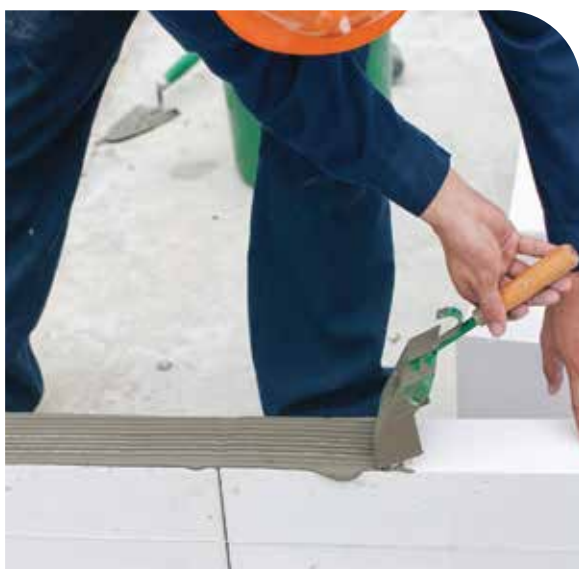
Applying thin-bed mortar using notched trowel enhances adhesive strength and saves material consumed.
