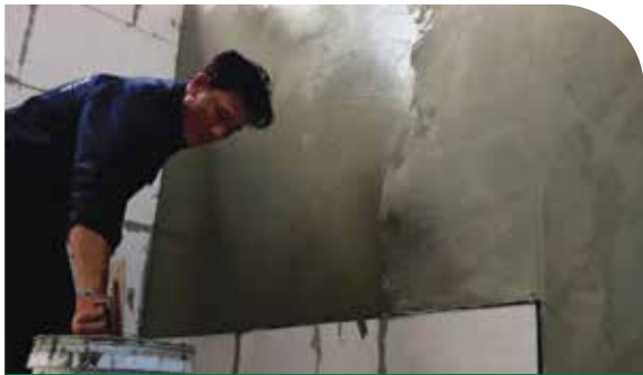
Skimcoat Mortar EBS-301 Application
